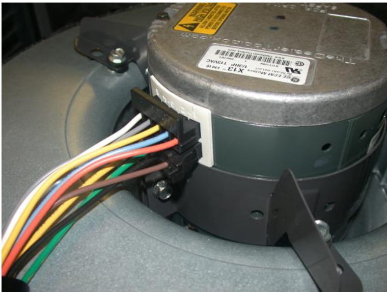
Figure 9 ECM-VE Motor Option- Control Box Connections
