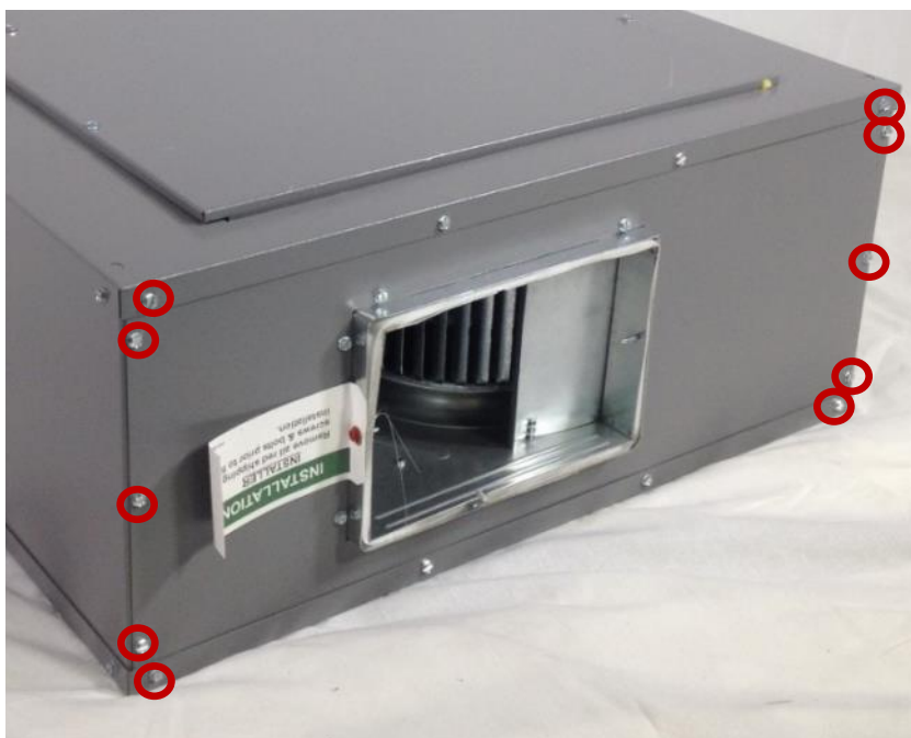
Fig 10 Remove indicated screws from front face sides
