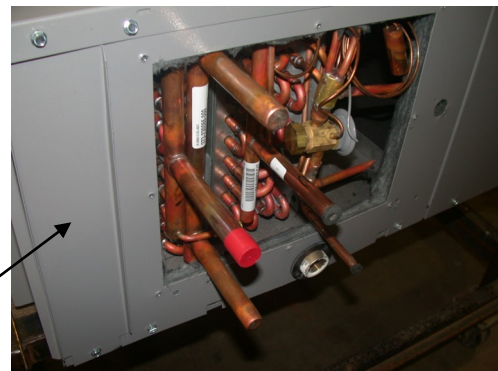
Figure 5 Coil Stubout Panel shown removed (sizes 04-20)
