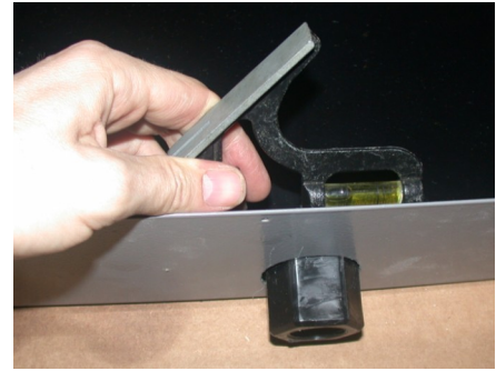
Figure 19 (level is resting on edge of plastic drainpan)
