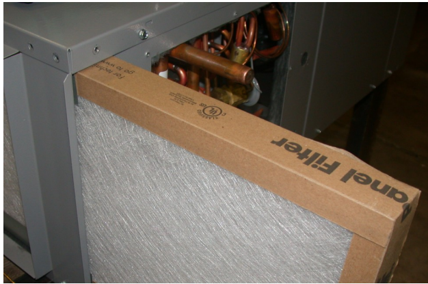
Figure 6 Filter removal.
